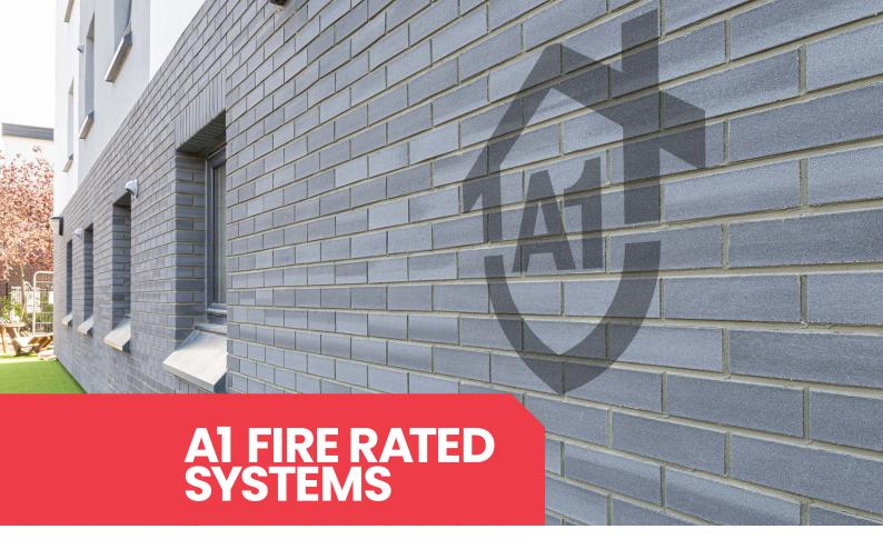
Most high-rise buildings typically require A2-s1,d0 fire rating according to European Classification to BS EN 13501-1. We have a range of **A1 systems** to exceed the requirements and offer the highest level of fire protection and non-combustibility.
