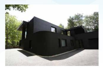
corners enabled the EPS insulation to flow continuously around the building, following the line of sub-structure.
