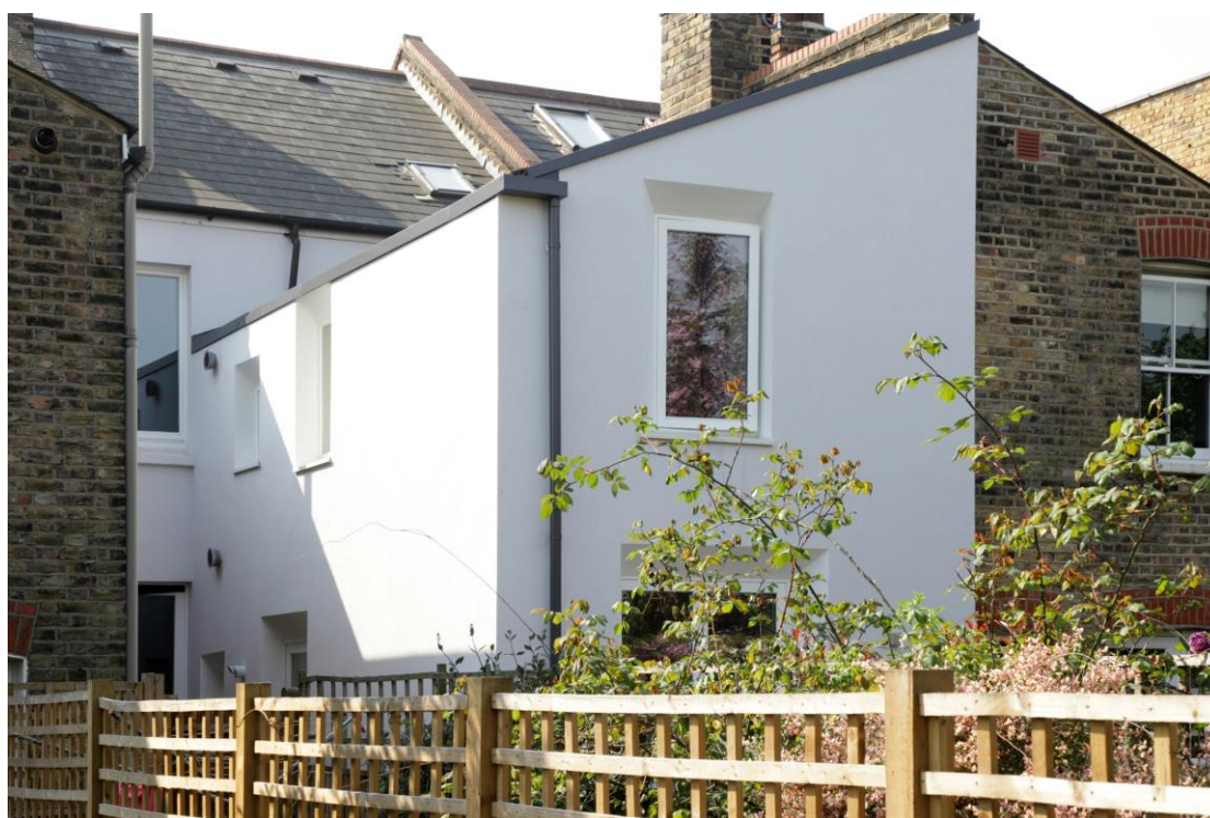
External insulation to a rear elevation
